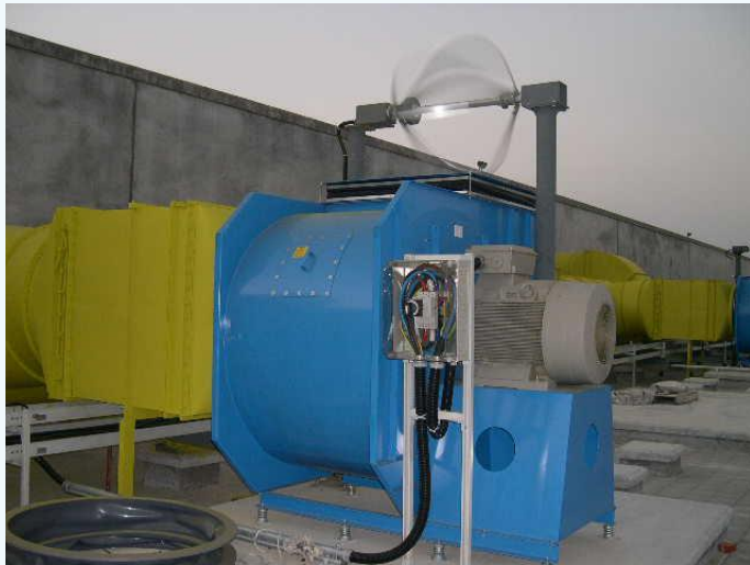
Installation of turbines for air extraction at AU Optronics corp. AUO in Taiwan
