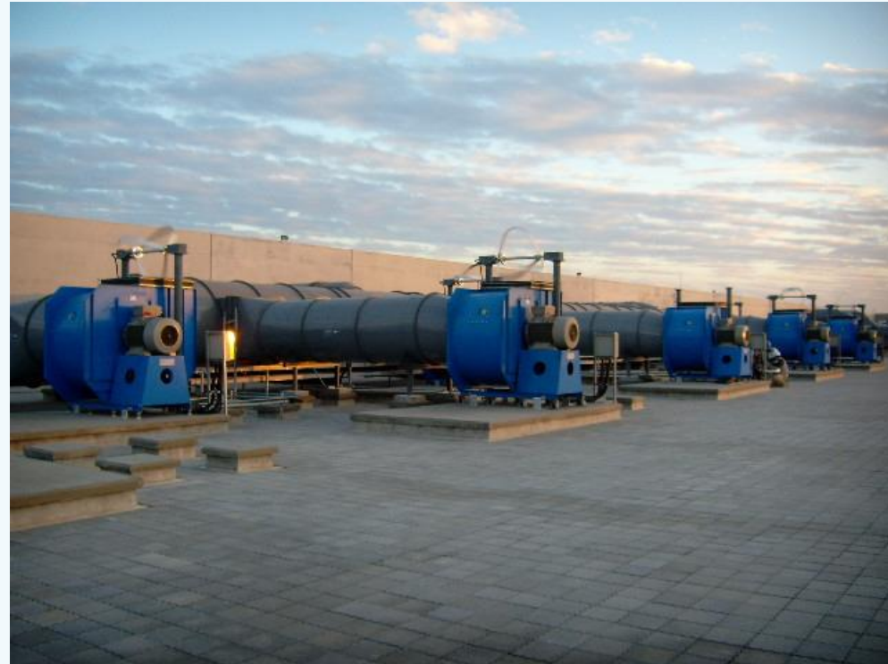
Installation of turbines for air extraction at AU Optronics corp. AUO in Taiwan
